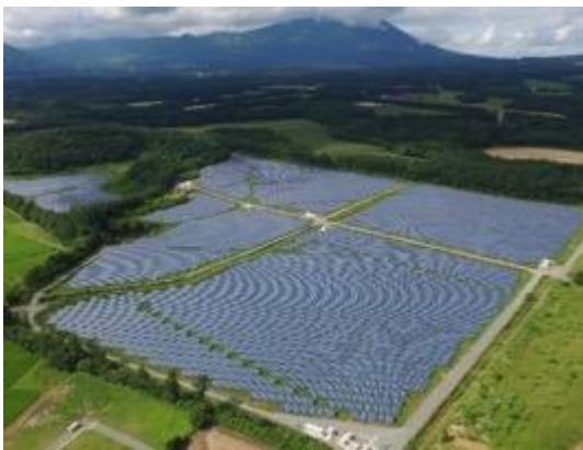
General aerial view of full plant
