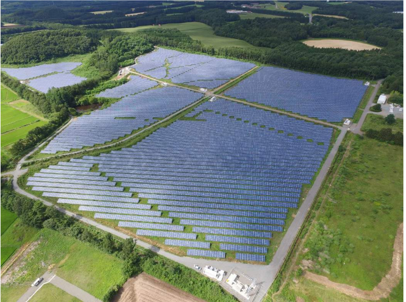
Shizukuishi solar power project in northern Japan
